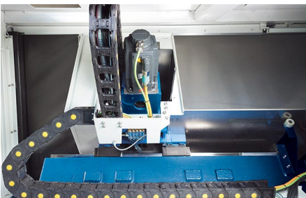
Siemens drive (here X-axis)
